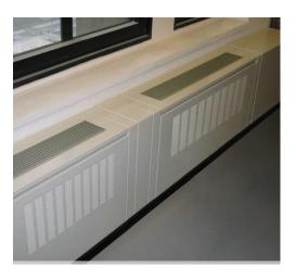
**Dual Air Streams:** Rittling Induction Units use two airstreams to maintain comfortable conditions. The primary air stream is delivered from central air handlers, while the secondary air stream is room air induced over the water coil within the unit.
